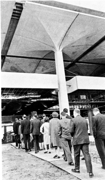
CONSTRUCTION PROGRESS —Touring ministers enter Dining Hall to view progress of building.
